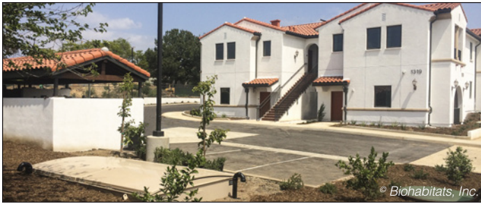
At Cedar Springs Apartments, high-quality effluent from an AdvanTex AX-Max™ is reused for toilet flushing and irrigation.
