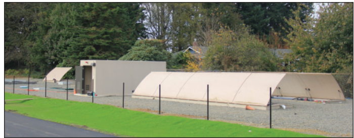
Irene Reither Elementary uses four AdvanTex AX-Max™ units and an Orenco DuraFiber™ Shelter in its nutrient-reducing WWTS.
