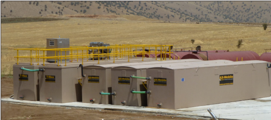
Portable AdvanTex AX-Mobile™ Wastewater Treatment Systems have been installed in remote areas of Kurdistan. They serve 500-person surveying camps.
