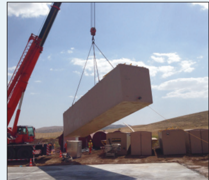
AX-Mobile units are completely pre-packaged and built inside a durable, insulated fiberglass tank that is easy to ship and set.
