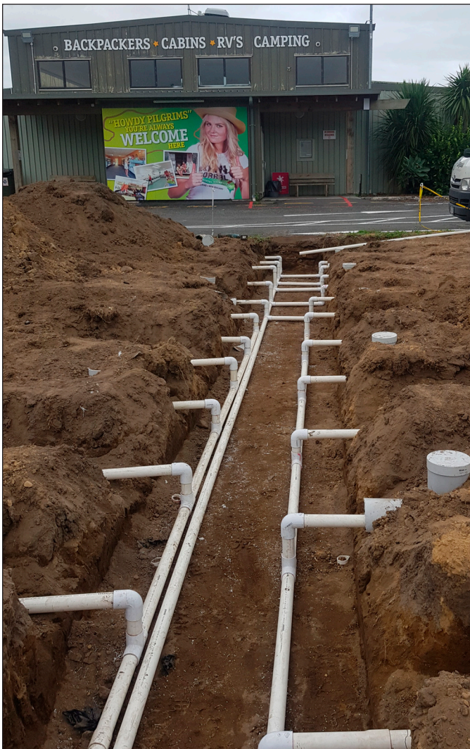
The use of this Orenco shallow pressurized dispersal system (SPDS) allowed for higher soil hydraulic-loading rates, which was necessary for Kiwi Corral's small dispersal field of just 430 m 2 (0.11 acres).
